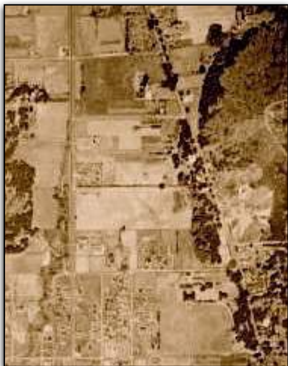
Aerial view of the neighbourhood in 1948. The empty fields at centre would be replaced by new houses within four years on Freeman, Veteran, St. Matthew's and Derby roads - the latter seen as a dark line of greenery across the middle. The so-called 'plantation' forest of the Whiteoak children lines the westside of Richmond Road on the right, above the University School (SMUS) campus.
